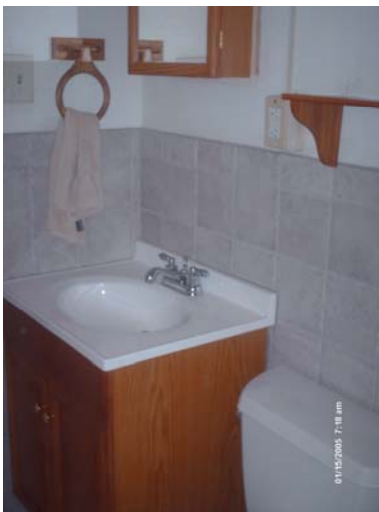
The bathroom in Phi's Suite was renovated by Brother Gallaher and his dad. What? No pink tiles!
